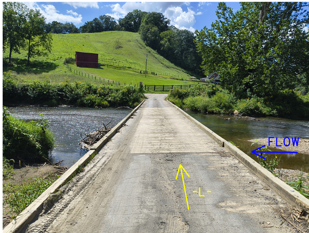
PHOTO #1: VIEW FROM END BENT NO. 1 FACING EAST TOWARD END BENT NO. 2.
