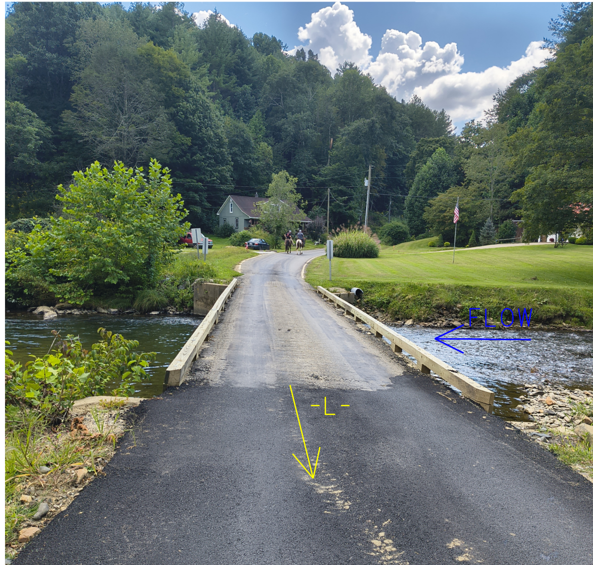
PHOTO #1: VIEW FROM END BENT NO. 2 FACING SOUTH TOWARD END BENT NO. 1.
