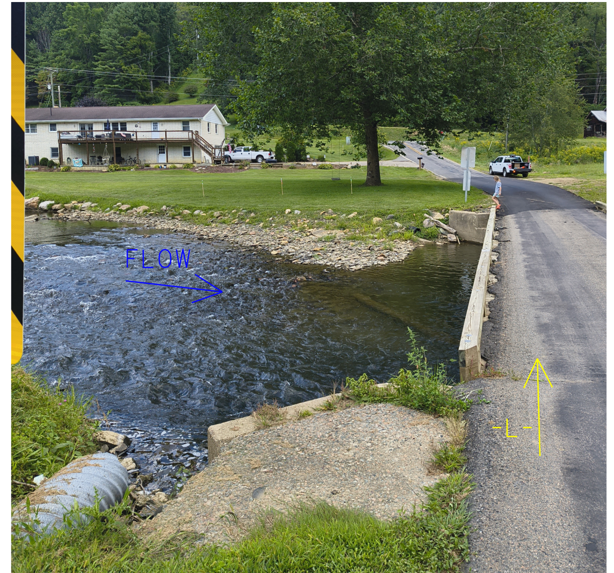
PHOTO #2: VIEW FROM END BENT NO. 1 FACING NORTH, UPSTREAM.
