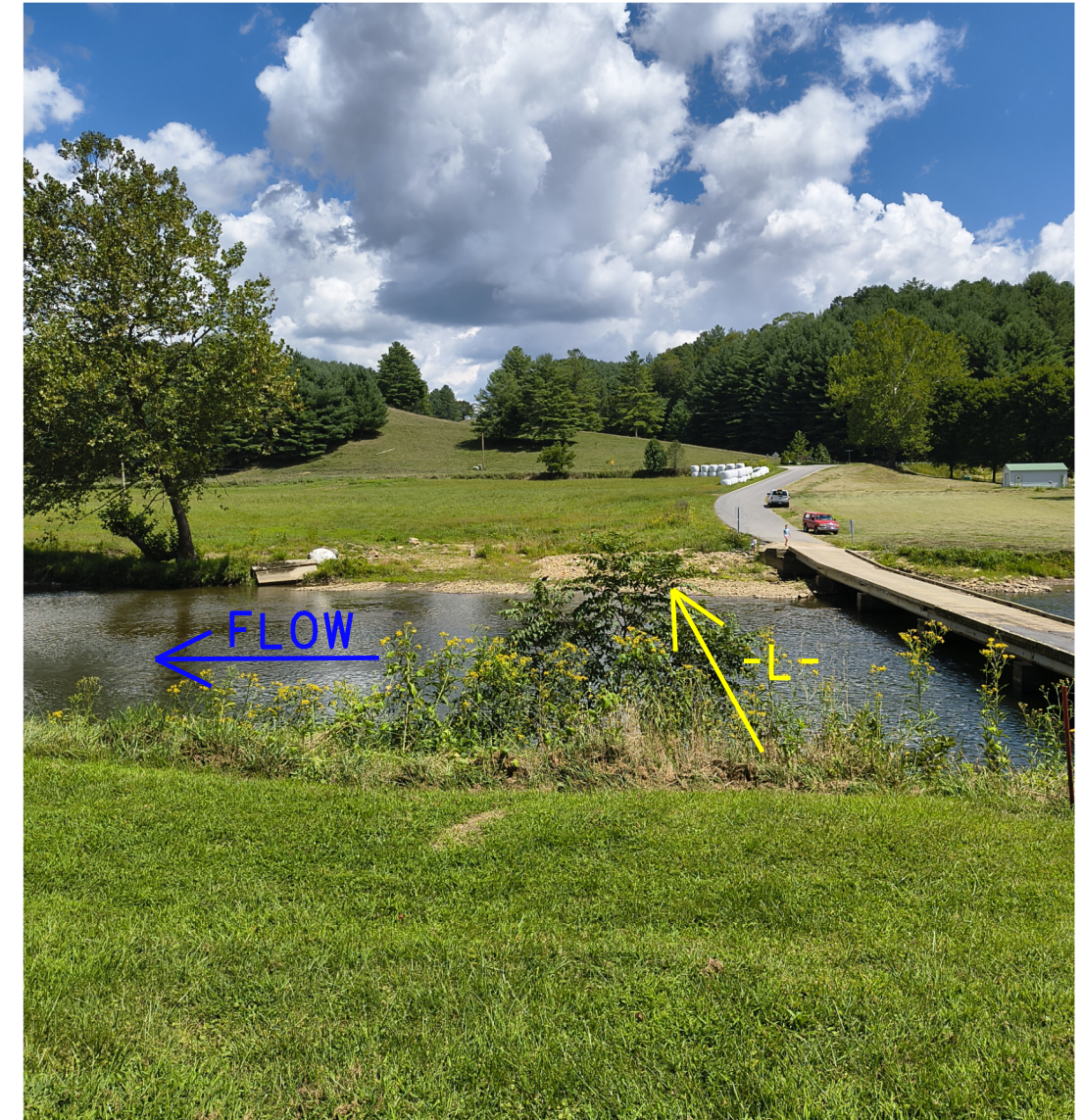
PHOTO #2: VIEW FROM END BENT NO. 1 FACING EAST TOWARD END BENT 2.
