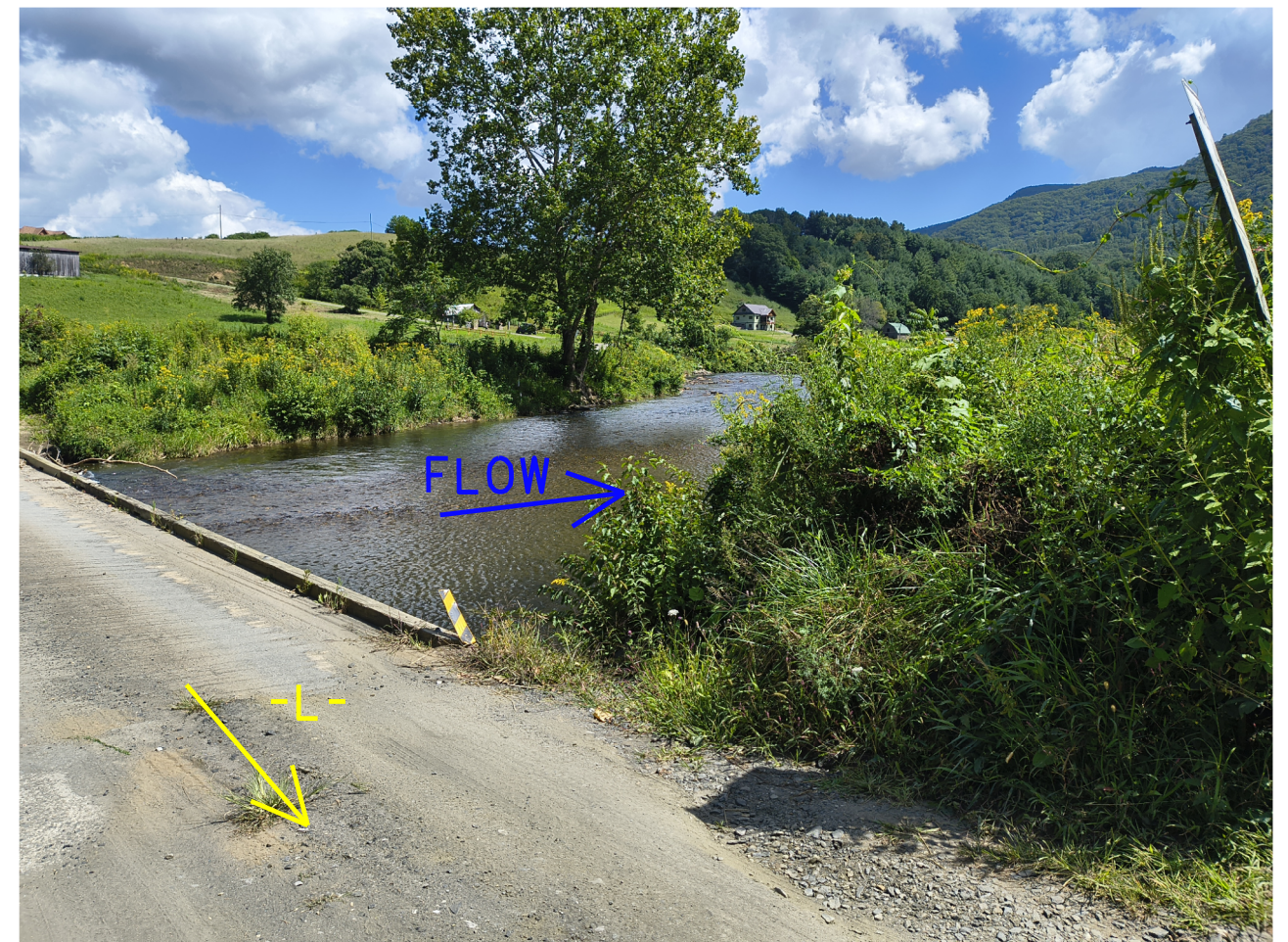
PHOTO #2: VIEW FROM END BENT NO. 2 FACING NORTH, DOWNSTREAM.
